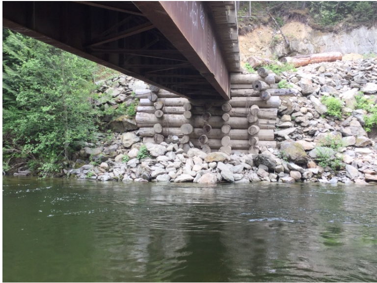
Right Bank Abutment when facing downstream
