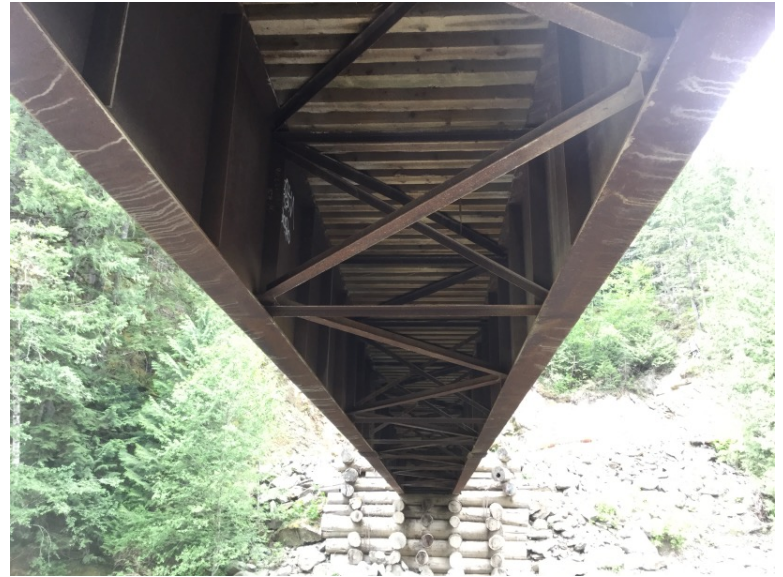
Main span Superstructure
