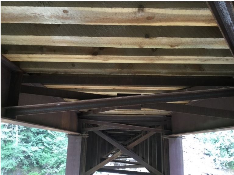
Jump span superstructure
